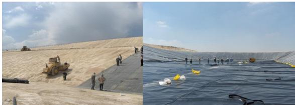
Figure 3.2: Lining of ZA L, (Source: JSC,2009).
